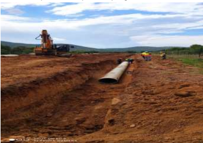
Laying of pipeline from Loskop to Pump station 1
