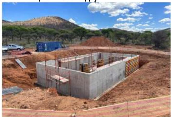
Pump Station 1 Concrete to Walls & Columns
